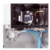
The INDUSTRIAL DRY range features a fully integrated and complete air treatment module including a refrigerated air dryer and both inlet and outlet high efficiency filters.
